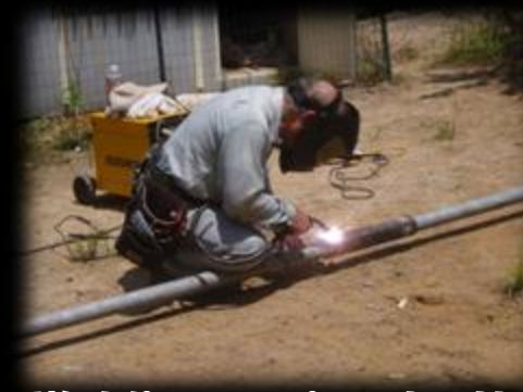
Welding a pipe to the mast
